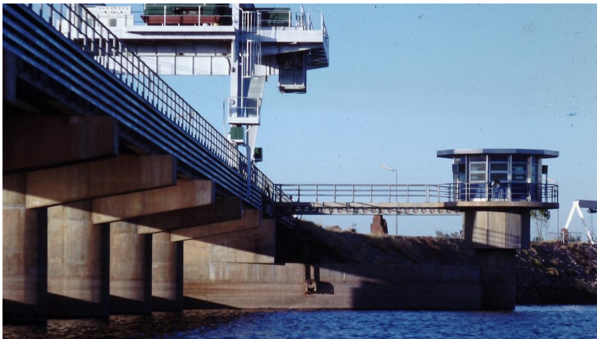
Figure 20: The diversion dam 1963 showing control tower and gantry crane
